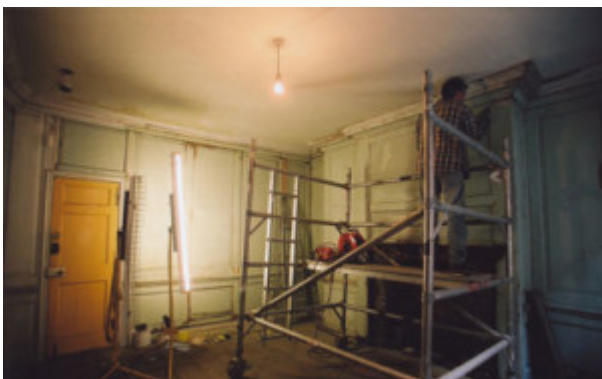
Fig. 6. Restoration of the interior.
