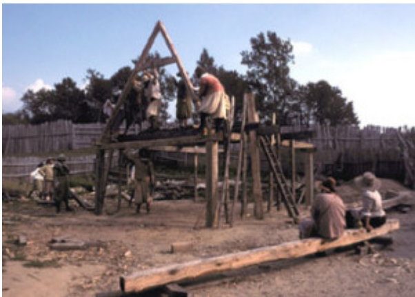
Fig. 1. The carpenters at Plimoth Plantation raise a house at their museum that is similar to the homes they would later build for the set of Colonial House . Photo by Emerson Baker.
